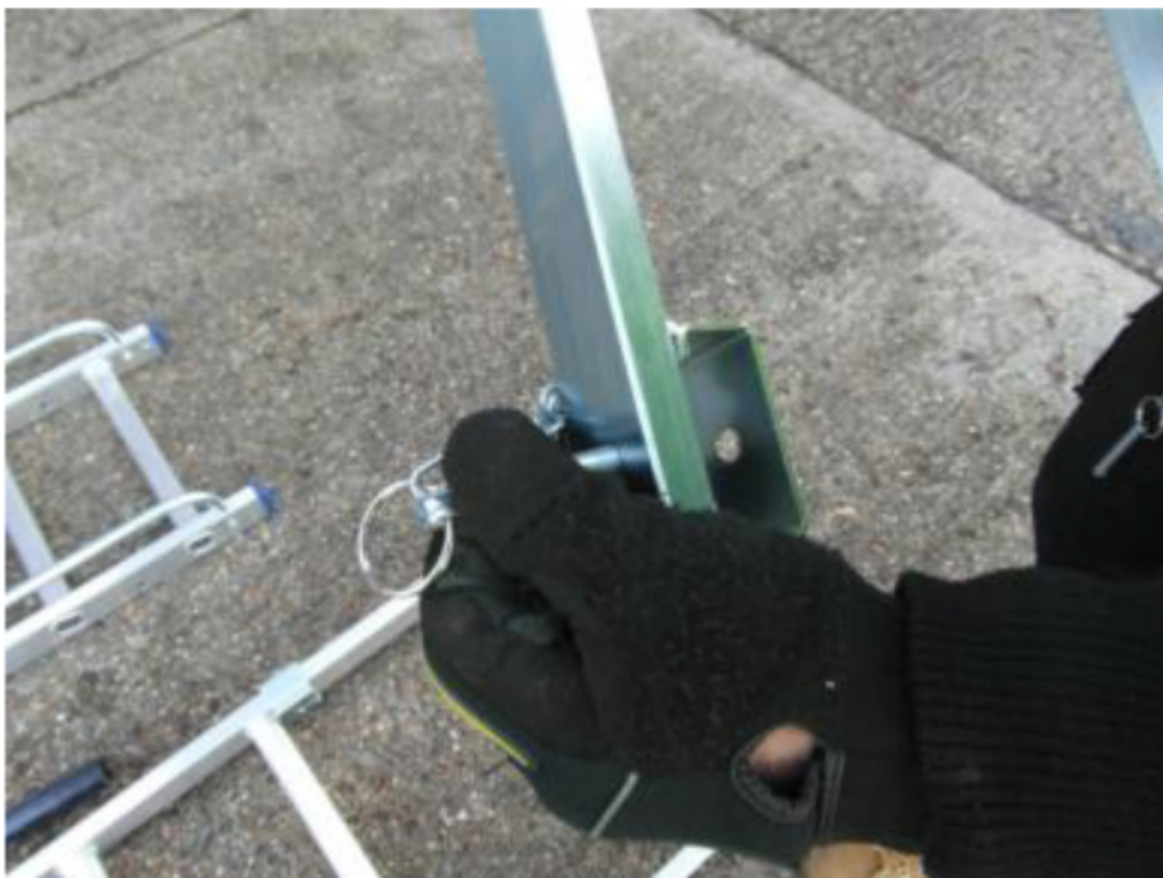
Remove the pins from the Eaves batten.
